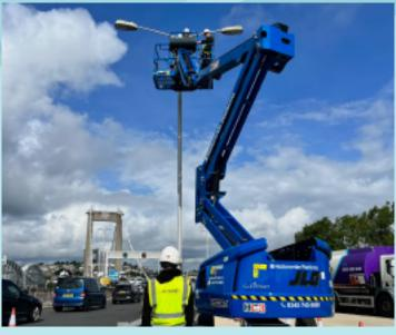
The firm returned to fit new, more modern, LED aircraft warning lights to the top of the towers 25 years ago. This time the main problem was finding the right size of brackets to fit the replacement lights to the towers.
